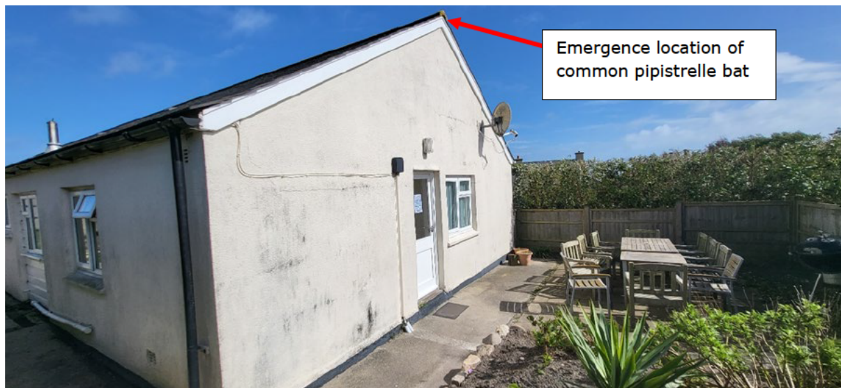
Figure 10: South elevation of Bottom Annexe. The red arrow indicates the emergence location of the single common pipistrelle bat during both surveys (18 th May and 22 nd June 2023)
