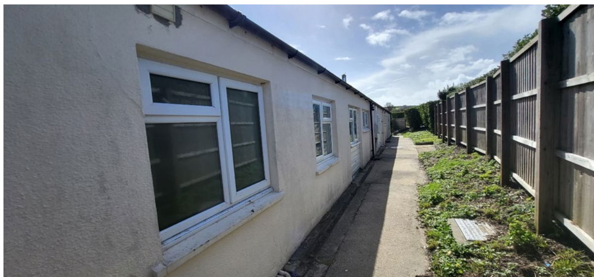
Figure 5: View of the west elevation of Bottom Annexe
