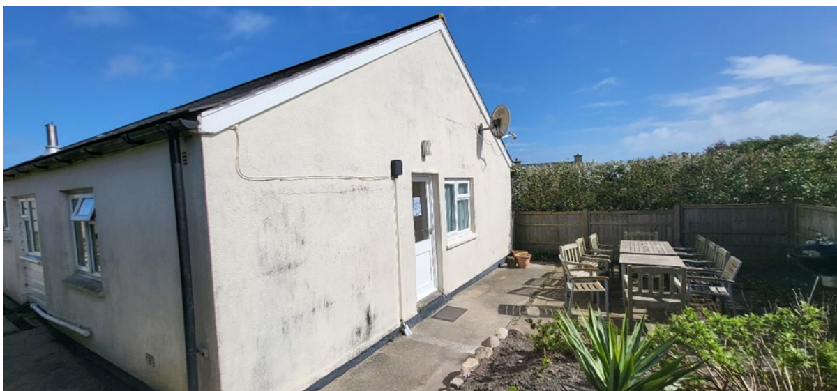
Figure 7: View of the south elevation of Bottom Annexe
