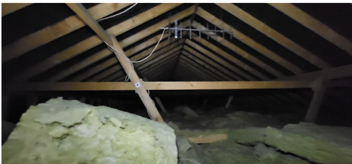
Figure 8: Interior of roof void 3
