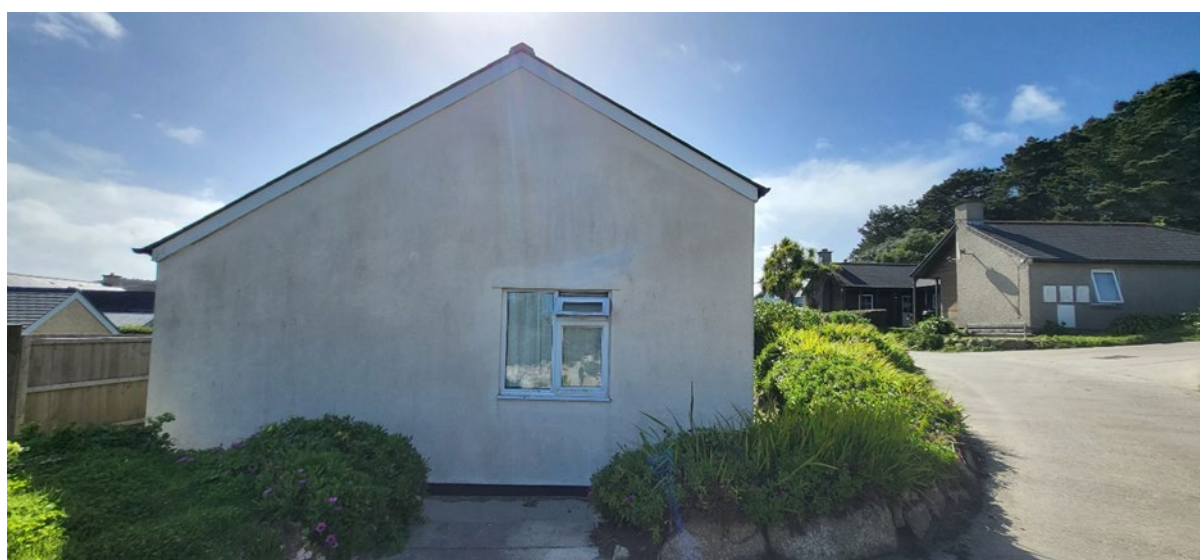
Figure 6: View of the north elevation of Bottom Annexe
