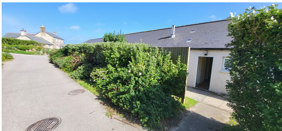
Figure 2: View of the west elevation of Bottom Annexe
