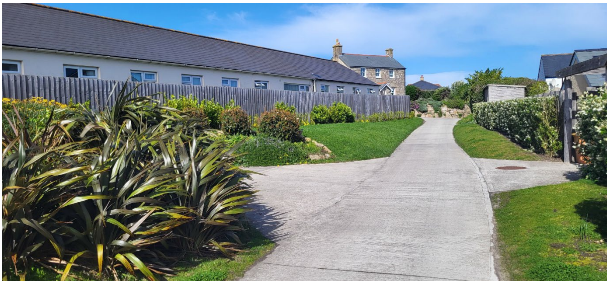
Figure 1: View of the east elevation of Bottom Annexe
