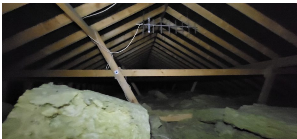
Figure 8: Interior of roof void 3
