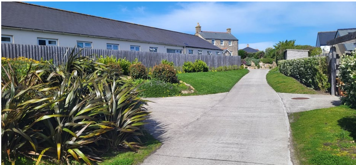
Figure 4: View of the east elevation of Bottom Annexe
