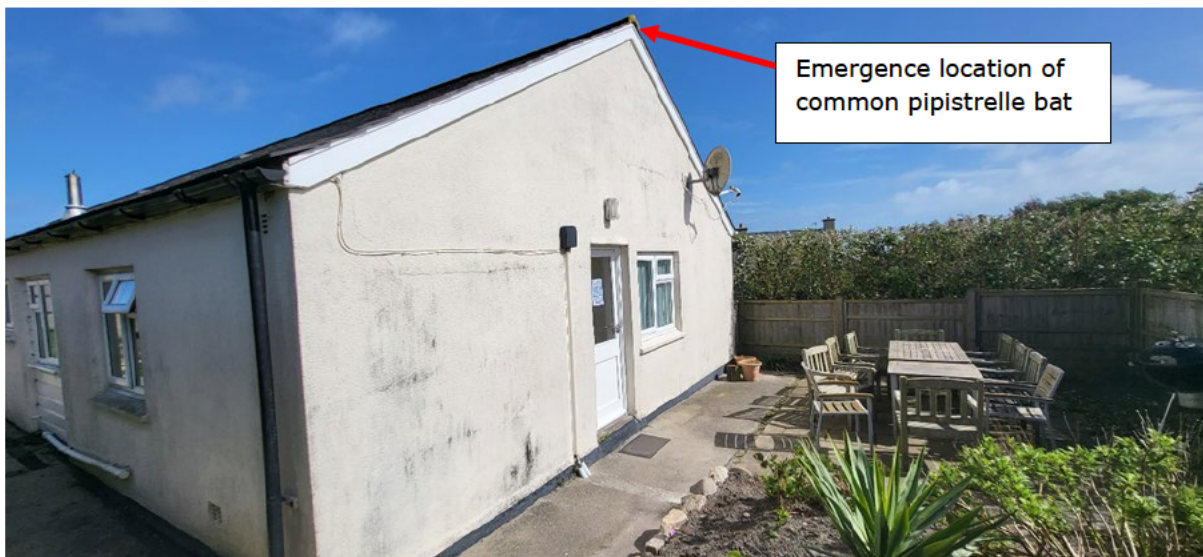
Figure 10: South elevation of Bottom Annexe. The red arrow indicates the emergence location of the single common pipistrelle bat during both surveys (18 th May and 22 nd June 2023)
