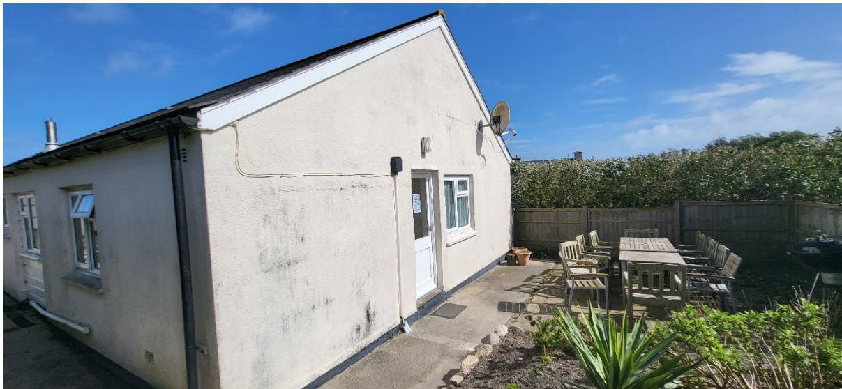
Figure 5: View of the south elevation of Bottom Annexe
