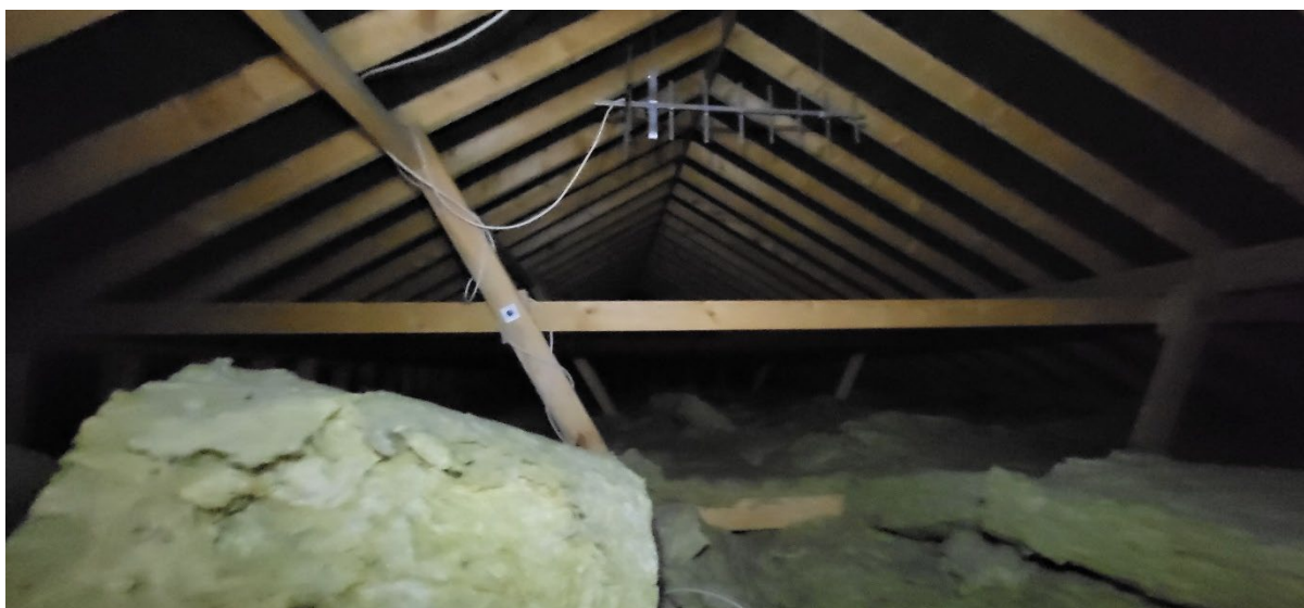
Figure 11: Roof structure of void 3. Bitumen roofing felt and timber frame
