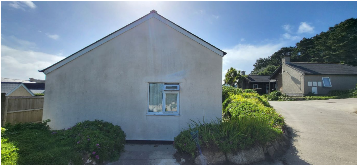
Figure 4: View of the north elevation of Bottom Annexe
