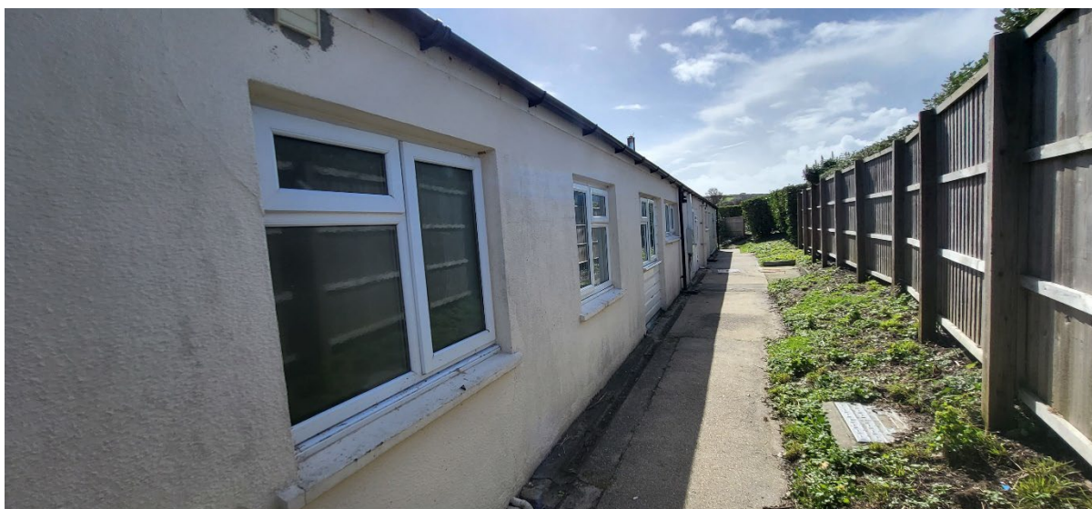
Figure 3: View of the west elevation of Bottom Annexe
