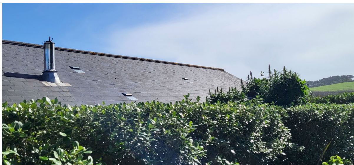
Figure 6: View of the flue and vents on the roof of the west elevation
