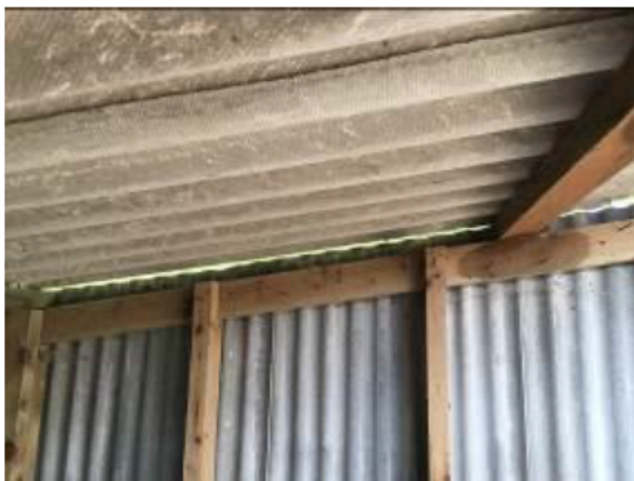
Photograph 3: Showing the upper wall and roof structure.
