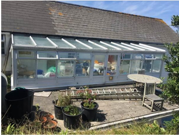
Photograph 1: Showing the conservatory (Section B) attached to the southern aspect of the main building (Section A)
