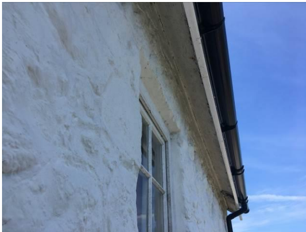
Photograph 3: Showing the well-fitted soffits supporting guttering on the southern aspect of the main building (Section A)
