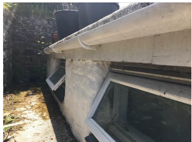
Photograph 6: Showing the fascia and guttering below the flat-roof section of the building (Section C) with well-fitted uPVC windows visible.
