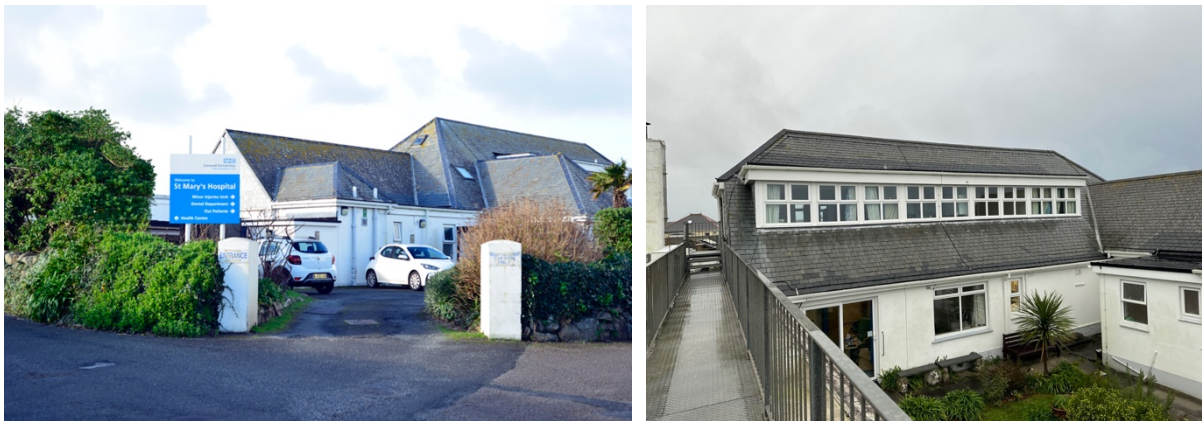
Figure 5&6: The Hospital entrance and from the rear
