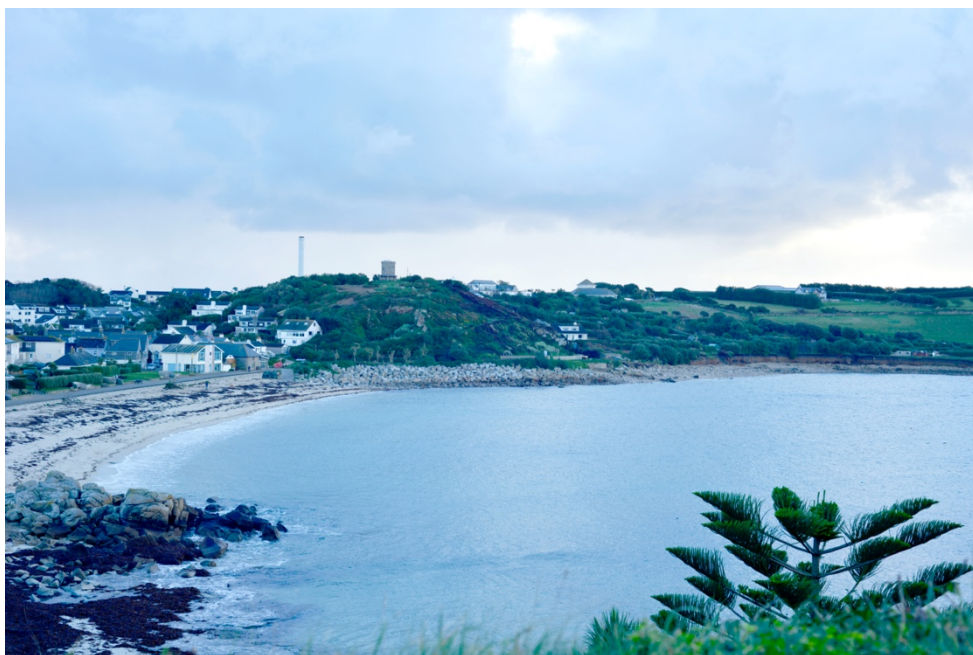
Figure 7: View across Porthcressa Beach towards Buzza Hill, the hospital and health centre.
