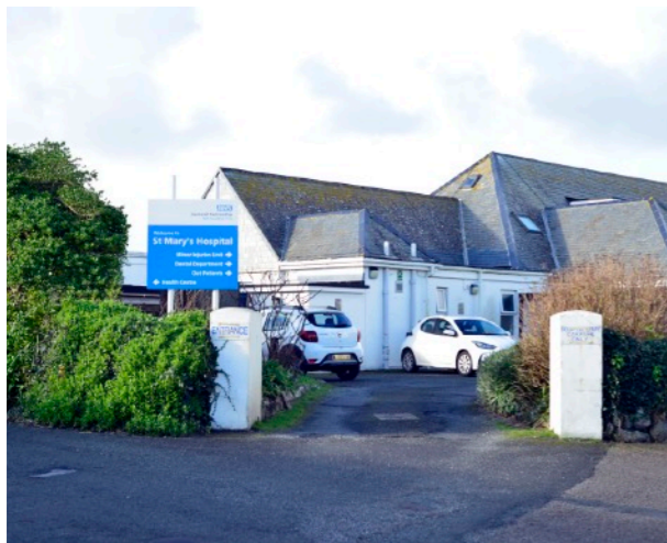
The existing site entrance
