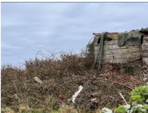
Photo 05 – Showing the wooden shed and surrounding bramble scrub.
