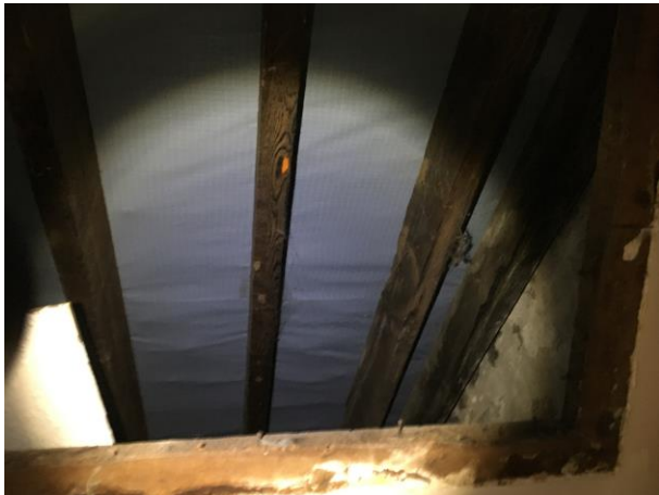
Photograph 9: Showing the roof structure within the minor loft space of the Extension.
