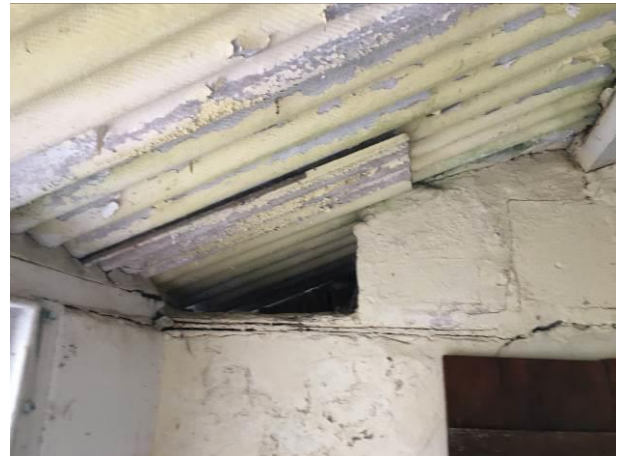
Photograph 10: Showing the interior of the Utility area.
