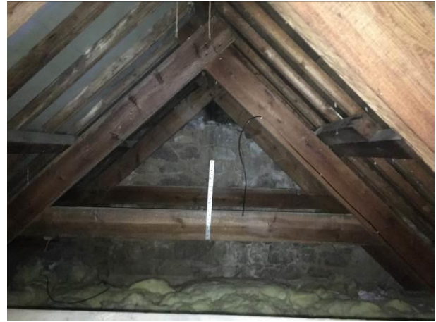
Photograph 8: Showing the interior loft space of the main Cottage
