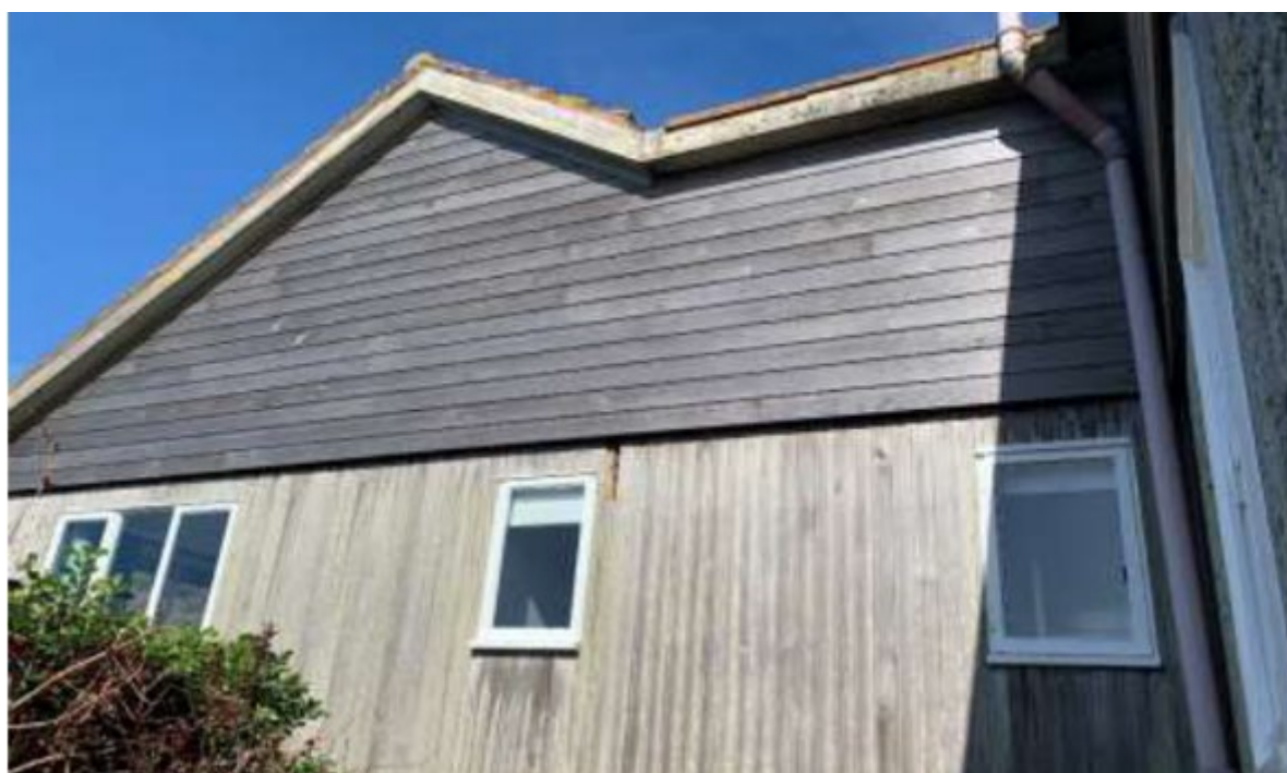
Figure 13: South elevation of Racket Town
