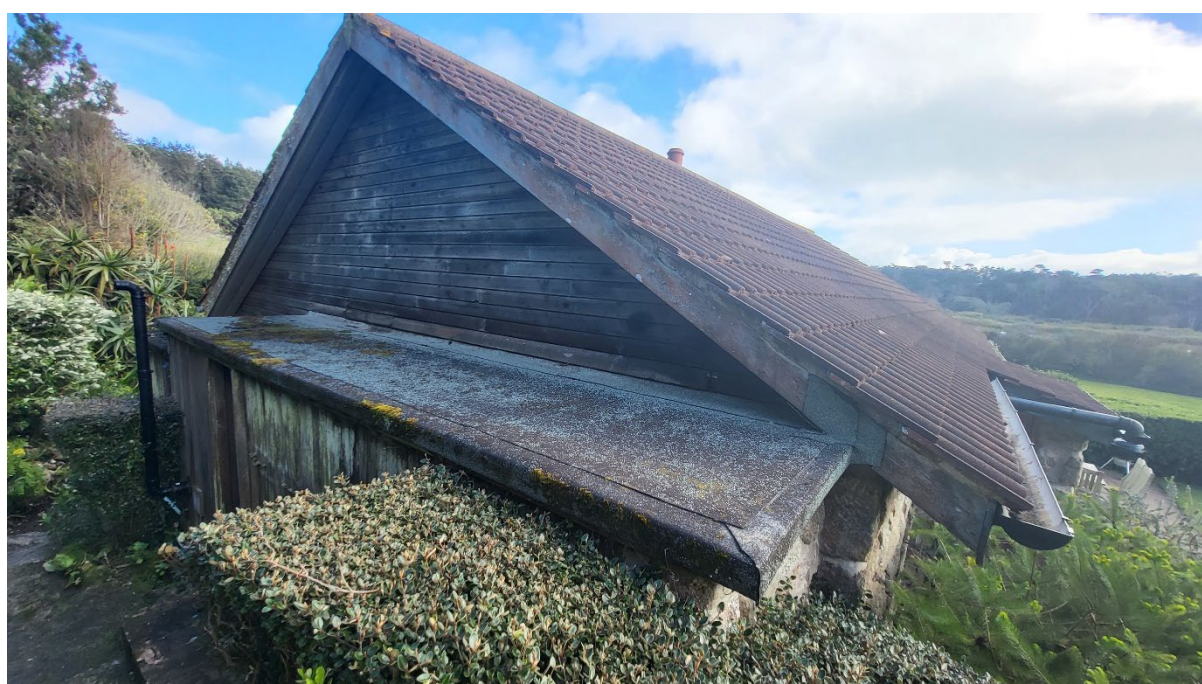
Figure 17: North elevation of Racket Town
