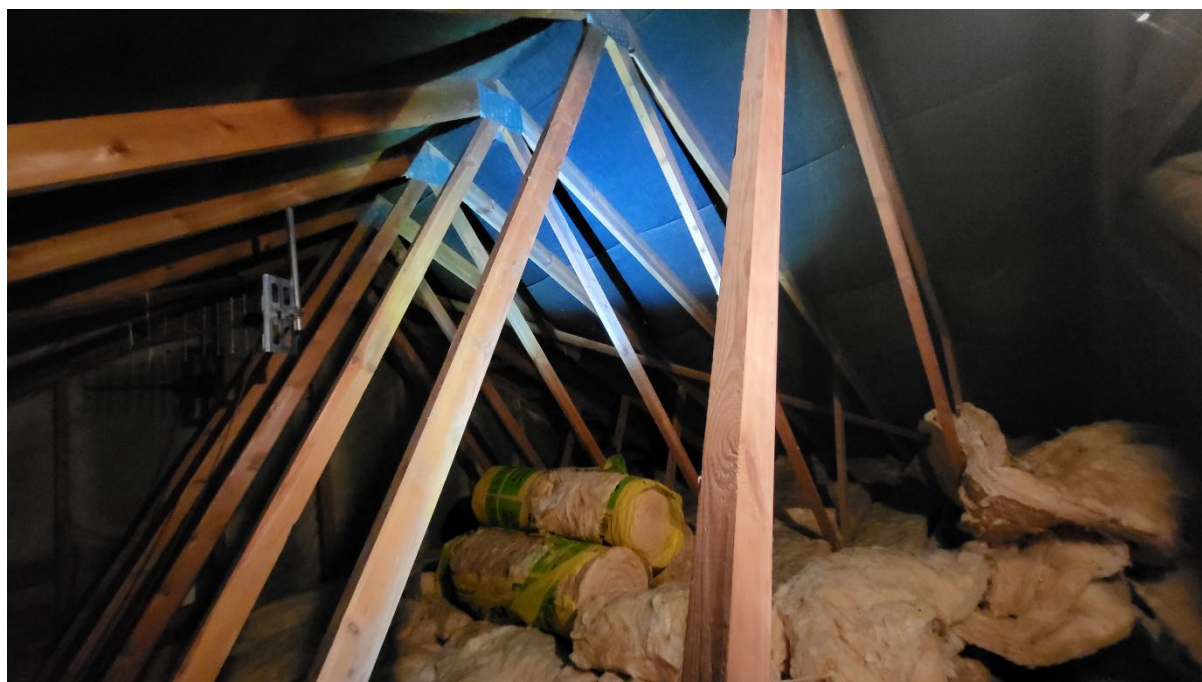
Figure 20: Interior roof structure of Racket Town with fink style roof truss
