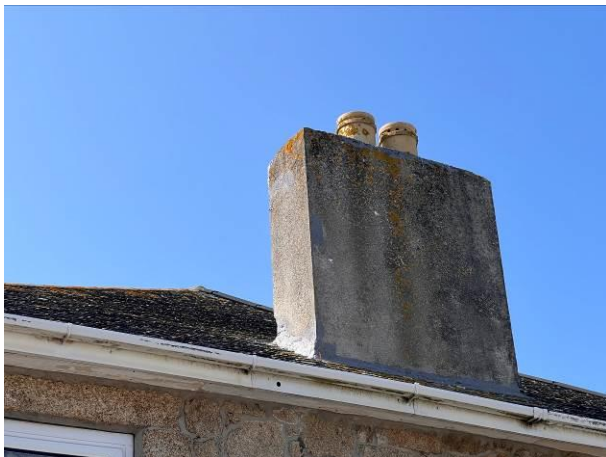
Photograph 3: Showing the rendered chimney to be removed
