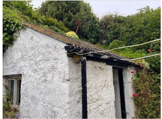
Photograph 8: Showing Outbuilding A with the fascia visible along the eaves. The well-sealed verge on the gable is also illustrated.
