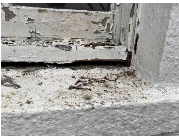
Photograph 3: Showing an example of the rot present in some window frames which does not yet offer roosting opportunities for bats but may develop in time.
