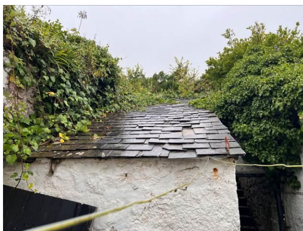
Photograph 6: Showing Outbuilding B with the natural slate tiled roof. The gaps between slates close to the eaves practise can be seen.
