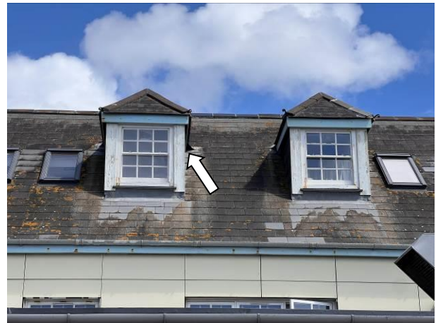
Photograph 4: Showing the main western aspect of Harbour B - the partially hipped dormers with sealed voids above can be seen. An example of the gaps in the flashing is indicated.
