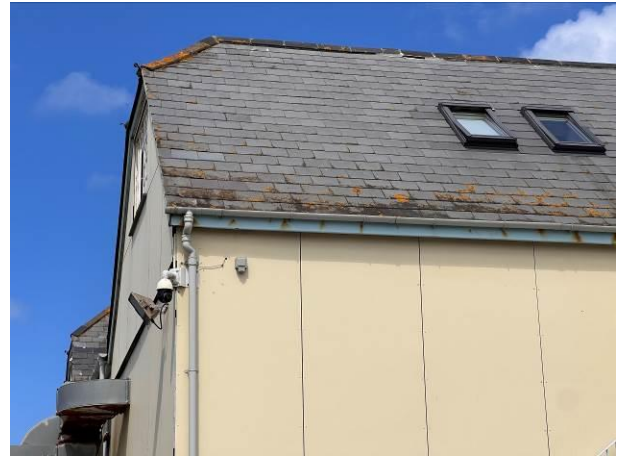
Photograph 2: Showing an example of the partially hipped roof structure of Harbour B with occasional roof lights within the span.
