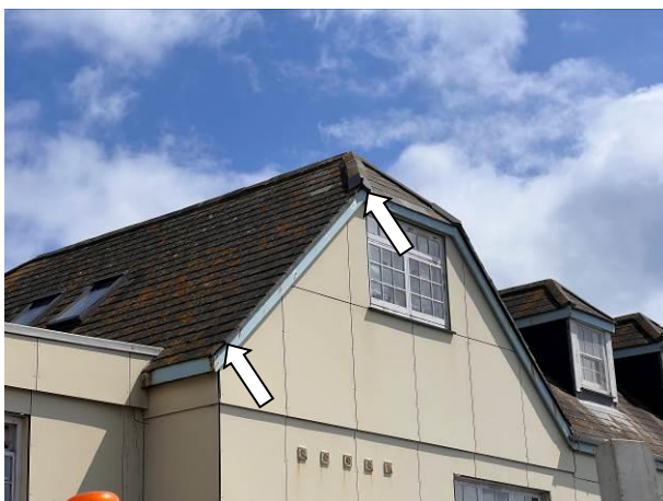
Photograph 5: Showing examples of gaps in the verge (LHS) and at the base of hipped ridge (RHS) on Harbour B
