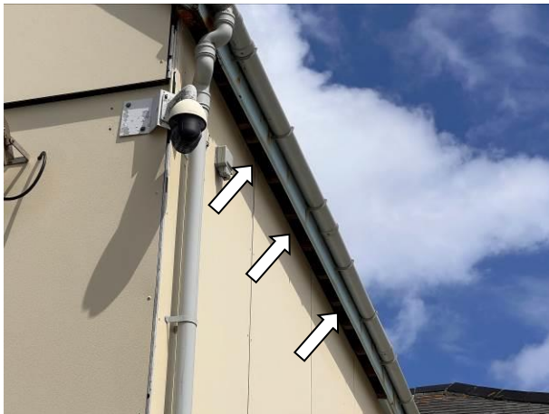
Photograph 3: Showing the gaps behind the damaged soffit on the northern eaves of Harbour B.
