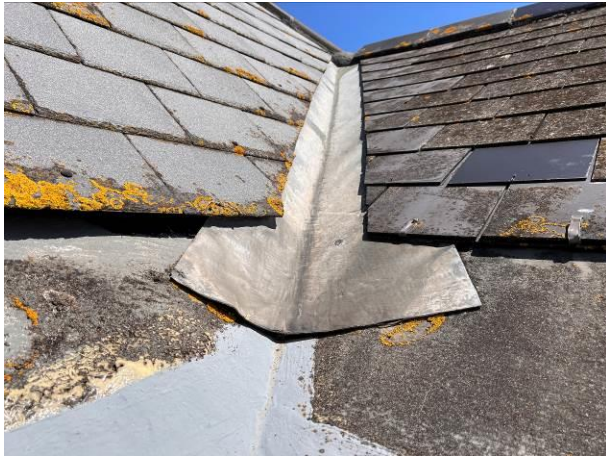
Photograph 7: Showing the typical roof structure within the roof-well of Harbour B – well-fitted synthetic tiles with well-fitted flashing are visible. Battens tightly fitted and present just above the termination of the tiles create a broad but superficial gap which does not have ideal dimensions nor fly-in access for use by roosting bats.
