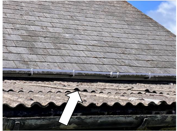
Photograph 8: Showing the gaps between overlapping corrugated sheets on the lean-to structure
