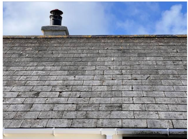
Photograph 4: Showing the tightly fitted roof tiles and ridge
