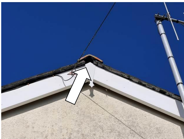
Photograph 5: Showing the gap under the terminal ridge tile at the gable. The gap behind the uPVC fascia below is too broad to provide suitable roosting dimensions for bats.
