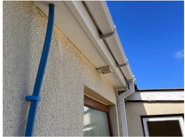
Photograph 2: Showing the uPVC soffit running along the eaves of the rear aspect of the main dwelling
