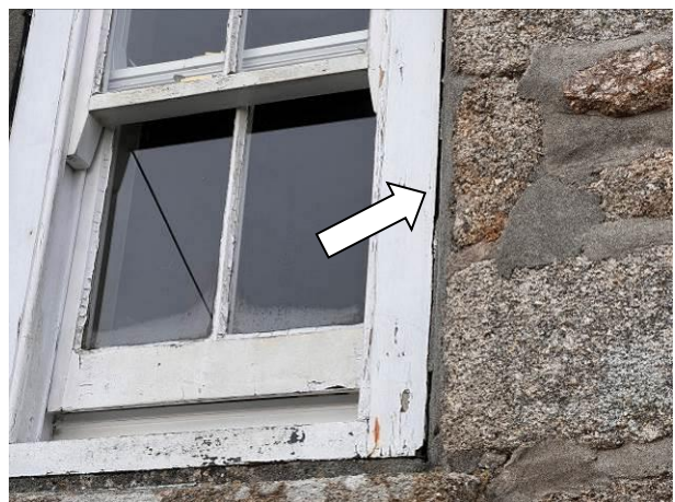
Photograph 6: Showing a window on the south-western aspect with minor gaps around the timber frame indicated.
