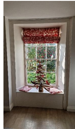
2. Existing internal shutter pocket (no shutter)
