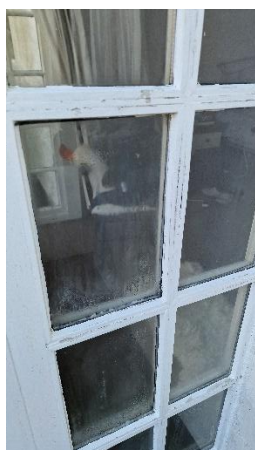
5. Existing door D- 01 – note interstitial condensation
