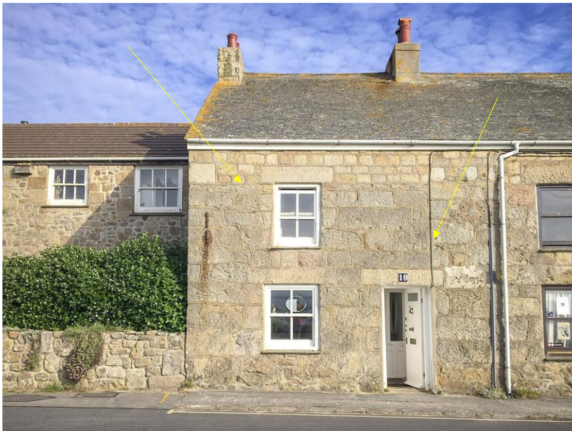
Pl.3: The front or north elevation of No.10 The Strand, construction breaks arrowed.
