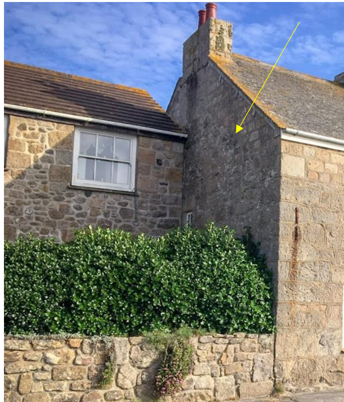
Pl.5: The east gable of No.10 The Strand, construction break arrowed.
