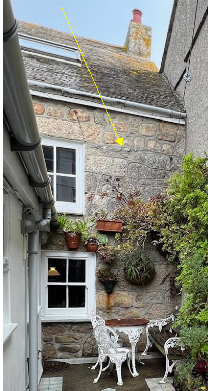
Pl.4: The rear or south elevation of No.10 The Strand, construction break arrowed.
