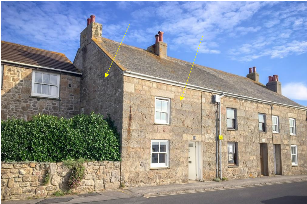
Pl.2: No.10 The Strand from the north-east with Nos.9 & 8 to the right. Breaks in the masonry showing original height arrowed.
