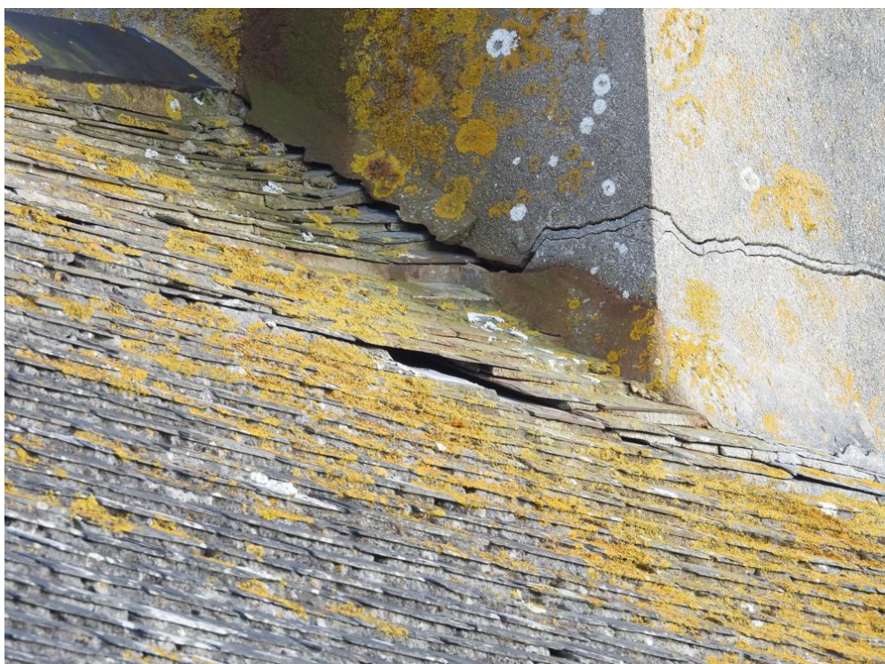
Pl.7: Detail of condition of the slating.
