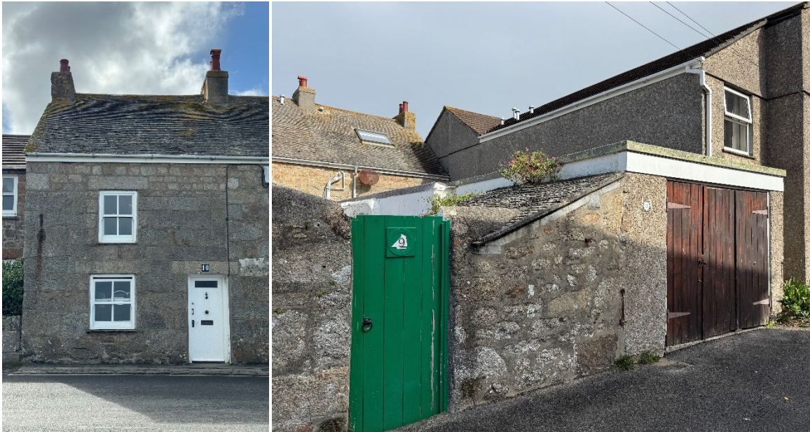
Front and rear elevation of property from Higher Strand (left) and Back Lane (right).
