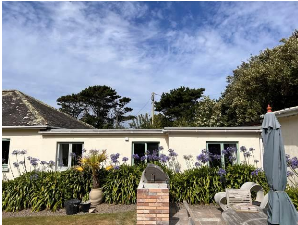
Photograph 1: Showing the flat-roof extension tied in with the bungalow on the LHS
