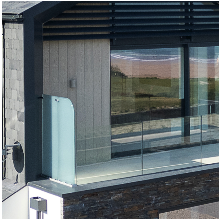
Condition C5 - Privacy screen Glass to be Pilkington Level 4 Height to be no less than 1.7m
