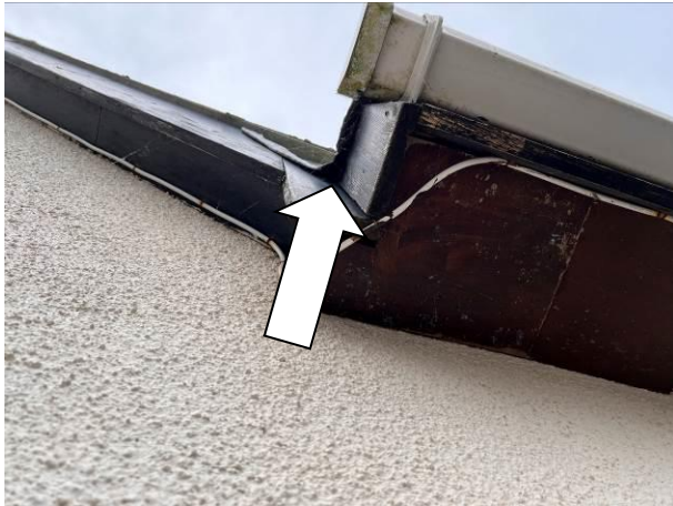
Photograph 3: Showing an example of the lifted flashing offering a potential roosting opportunity.
