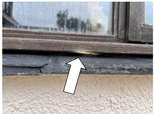
Photograph 6: Showing an example of a gap beneath a sill which was inspected fully.
