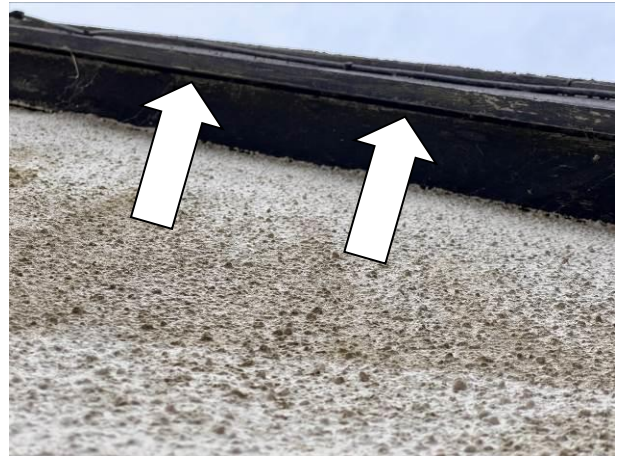
Photograph 4: Showing an example of a structural gap between the soffits on the western gable.
