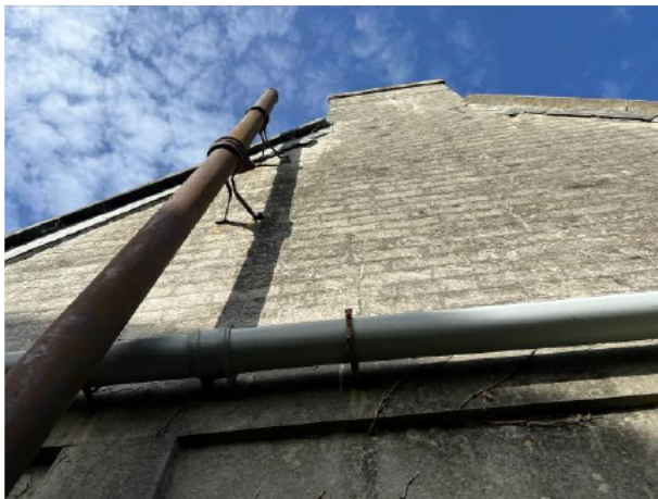
Photograph 3: Showing the southern gable of the property – there superficial gaps behind the drop-tiles on the eastern aspect can be seen on the right-hand side. Those on the western aspect would not be affected.
