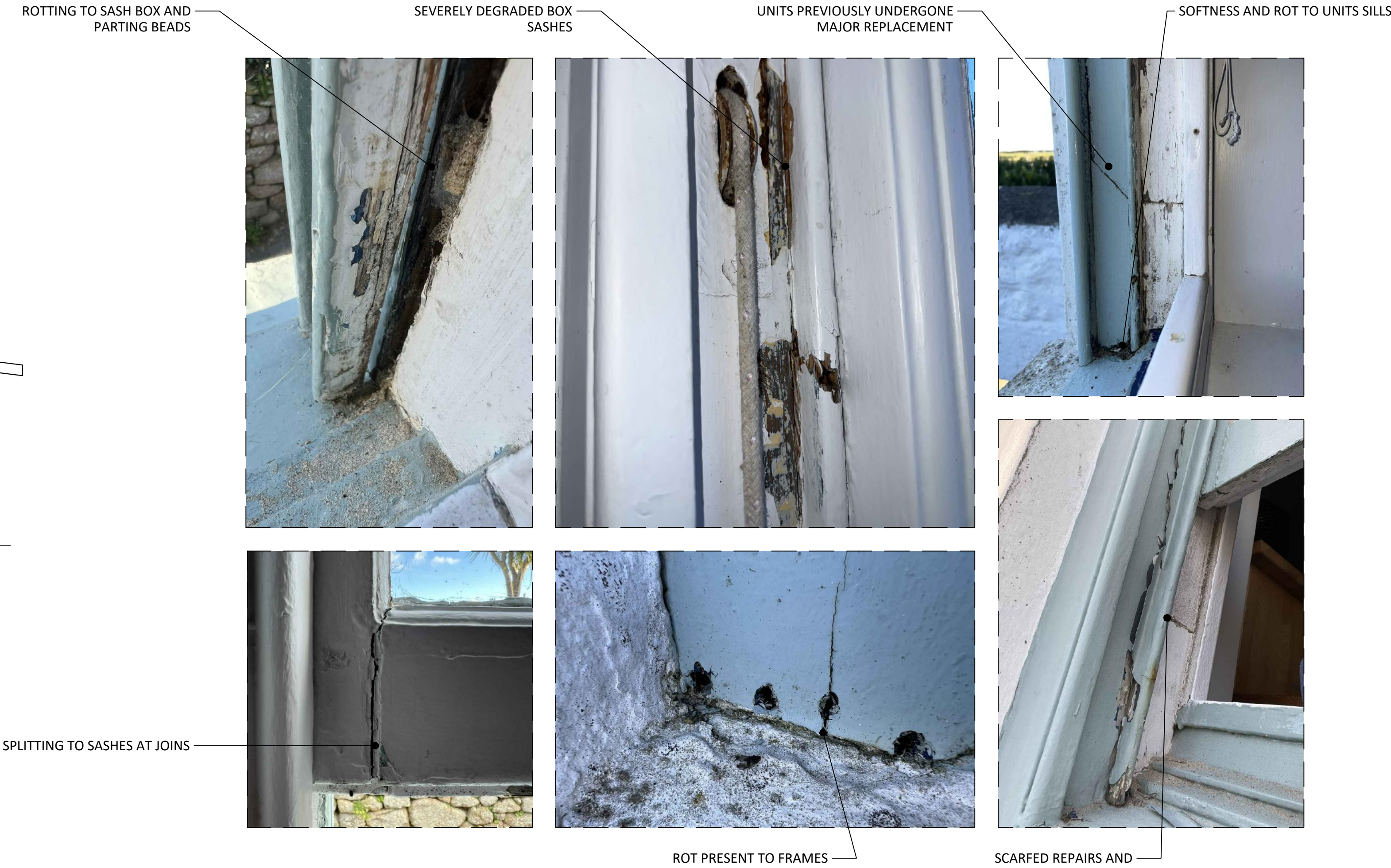
06 GROUP 1 TYPICAL DEFECTS REF 3528-1-500 SCALE N/A
