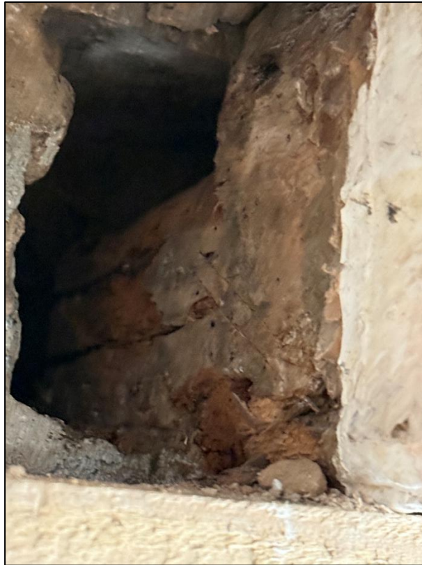
Exposed southern joist bearing showing some rot & longstanding decay.
