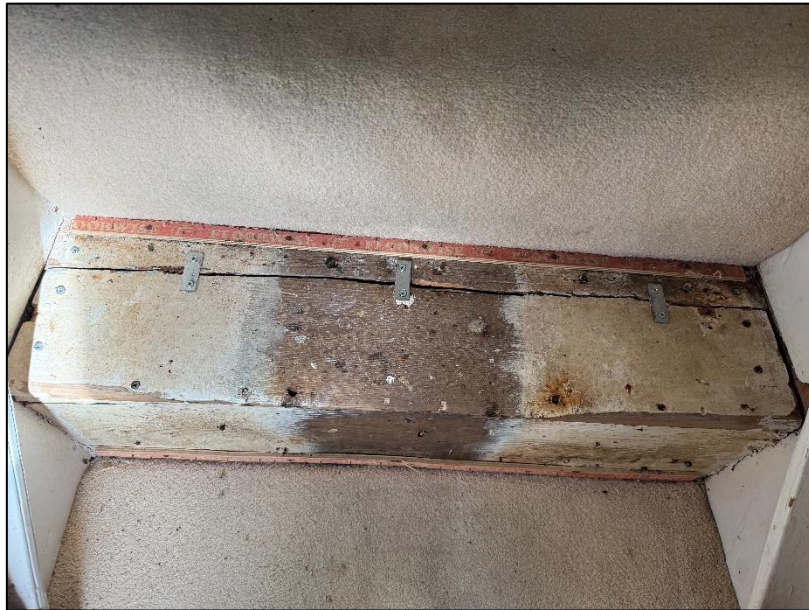
Split second tread requiring sympathetic repair.
