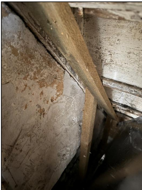
Current added support timbers under stair flight which would benefit from tidying & enhancing.
