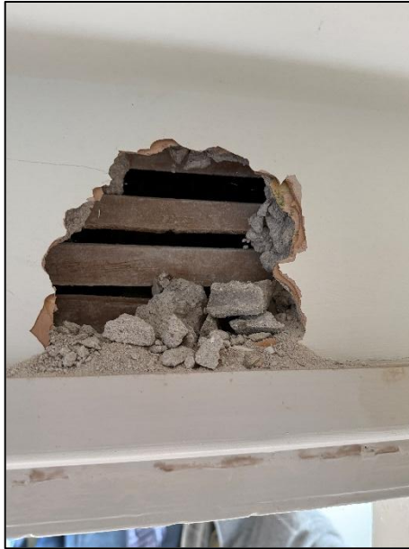
Investigation hole over dining room doorway showing timber lathes, with plaster overlaid with 12.5 plasterboard & skim.
