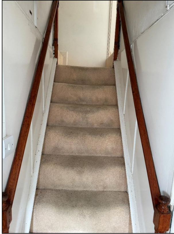
Existing original newel posts and handrailing to be adjusted and retained should a new 'over flight' be agreed.
