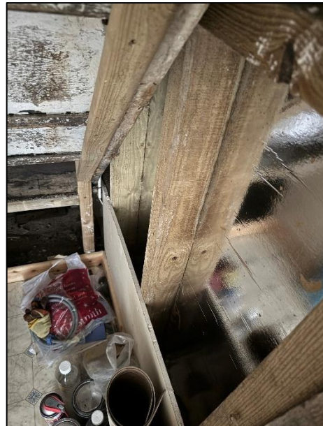
Current added support timbers under stair flight which would benefit from tidying & enhancing.
