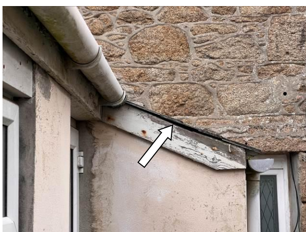
Photograph 5: Showing the gap in the verge on the single-storey extension where the footprint of the building extends out.
