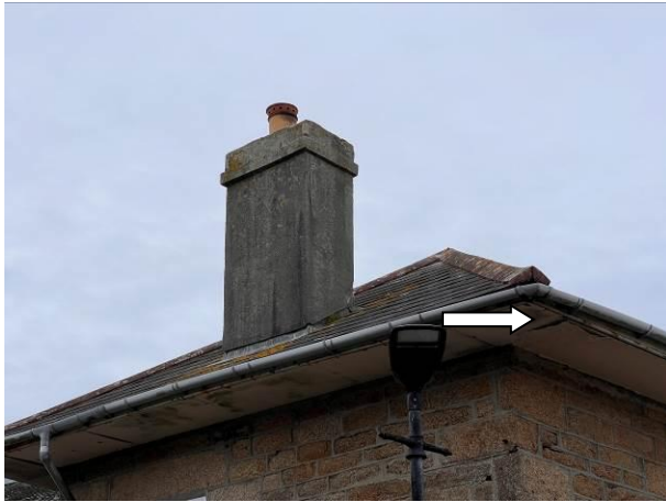
Photograph 7: Showing an example of damage to the soffit away from the junction with the main building wall.
