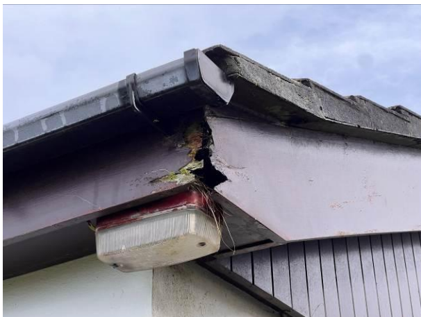
Photograph 5: Showing the gap in the soffit on the south-west corner of the property.
