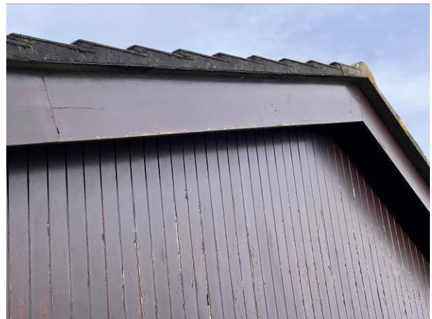
Photograph 4: Showing a closer view of the timber cladding and well-sealed soffit as well as the well-pointed verge on the gable.
