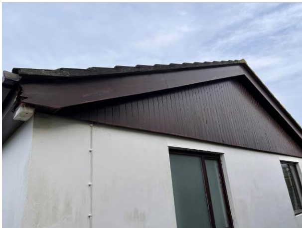
Photograph 3: Showing the gable end of the property with the soffit and vertical timber cladding.
