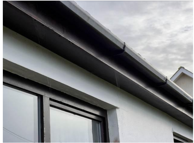
Photograph 2: Showing the well-sealed soffits of the property on the rear aspect.
