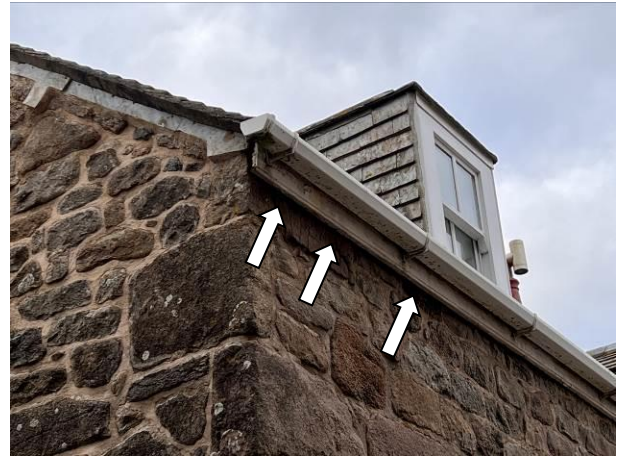
Photograph 2: Showing the dormer windows with hanging tiles on the north-eastern aspect of Pier House. Gaps beneath the fascia are indicated.
