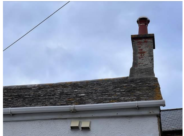
Photograph 4: Showing the south-western aspect of pier House with the well-sealed fascia and concrete-rendered chimney visible.
