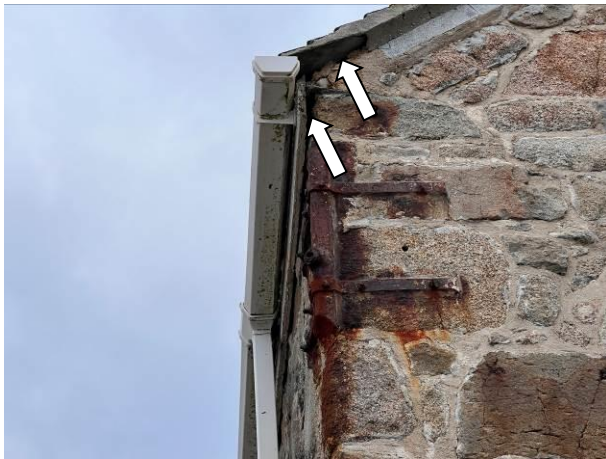
Photograph 3: Showing the gaps behind the north-eastern fascia and on the north-western verge of Pier House.
