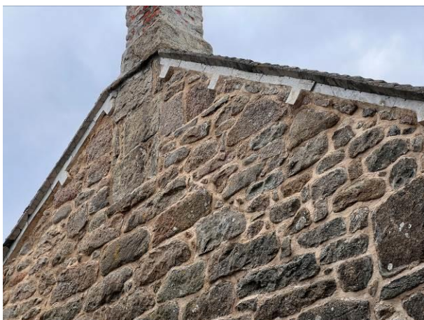
Photograph 5: Showing the south-eastern gable of Pier House with well-pointed drop tiles.
